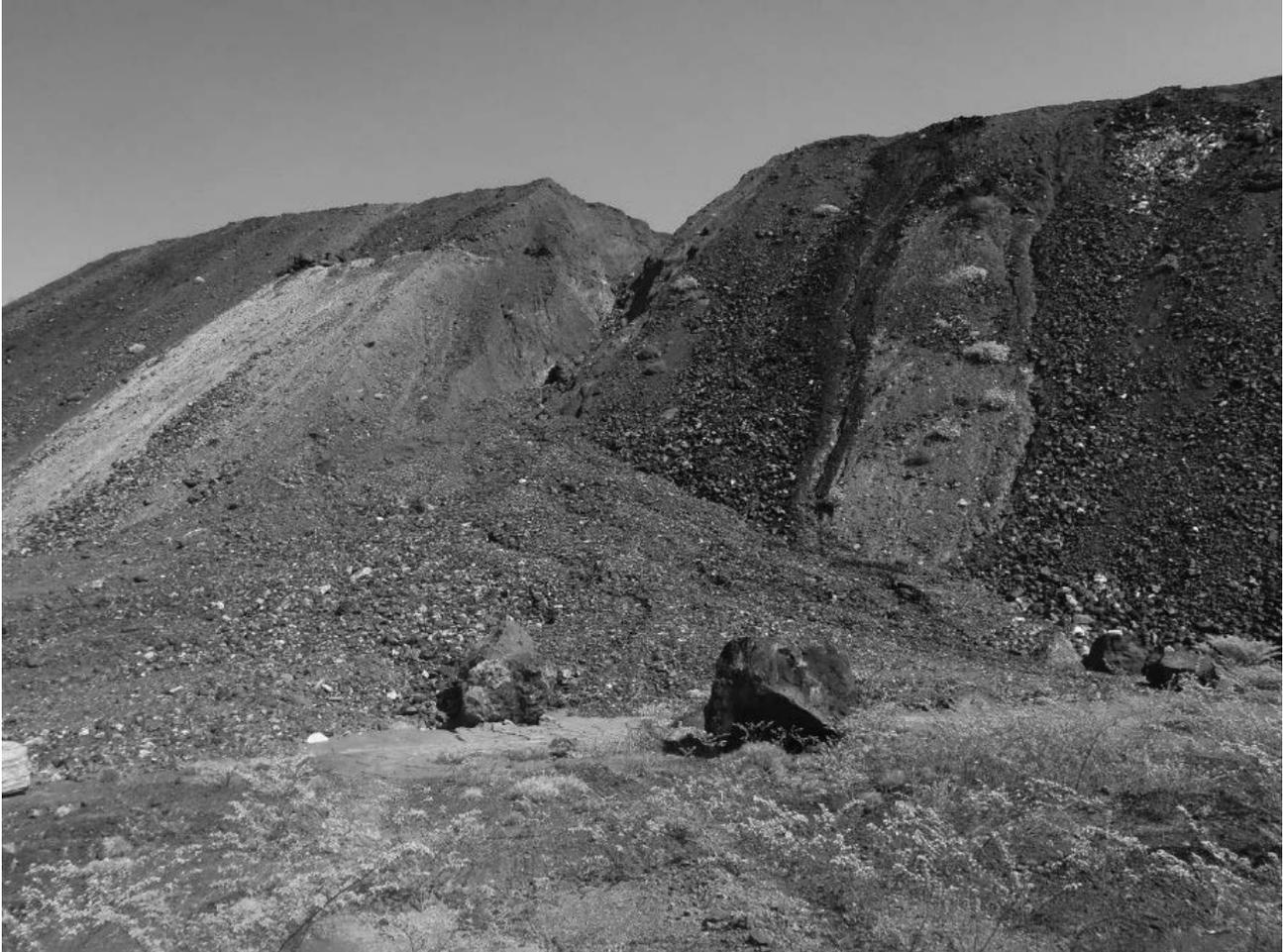
Figure 4 Erosive rock from a WRD where durable rock was predicted (Case study 2)
